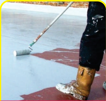
BASEMENT WATERPROOFING
